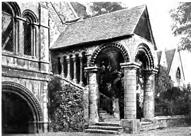
Fig. 2.—NORMAN STAIRWAY IN GREEN COURT.
